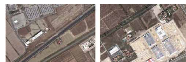
11. Two periurban areas analysed by the Lazio regional government show how the historic dimension of the landscape is no longer legible. These two aerial photos show how the relationship between the major transport infrastructure (left, in the Portuense area), the major territorial service infrastructure (right, in the Isola Sacra area) and the fabric built around the country houses remains unclear.
