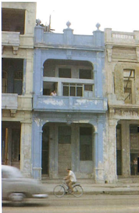
MALECON N° 27. RESTAURATION WORKS MALECON. HAVANA Malecon Project Cuba+Spain, Seville
